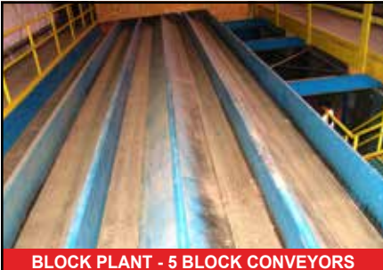
BLOCK PLANT - 5 BLOCK CONVEYORS
