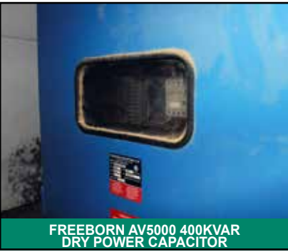
FREEBORN AV5000 400KVAR DRY POWER CAPACITOR
